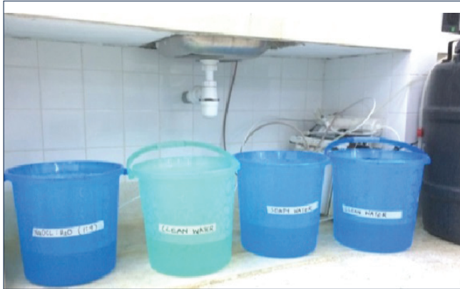
Bucket system for cleaning and decontaminating equipment before sterilisation (photo taken at Kwale).
