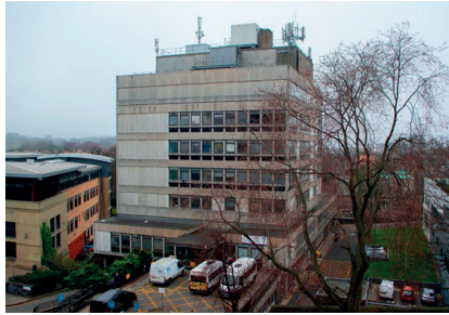
Figure 2: The PAEP building in 2019.
